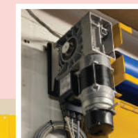
Motor 3 Phase 400v AC worm gear and brake motor (with anti roll back) Encoder switches for open and close positions. Adjustable opening and closing speeds Curtain barrel is driven by motor drive unit eliminating the need for chain drive
